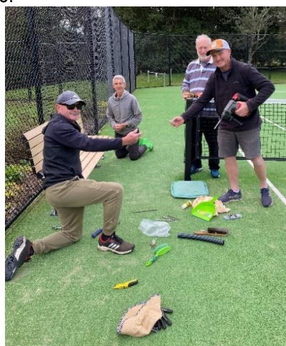
A happy bunch of installers at work.
