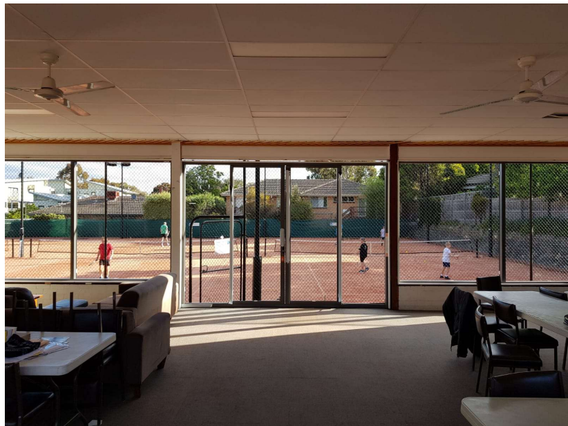
The new view after the replacement of all windows and doors and repainting.
