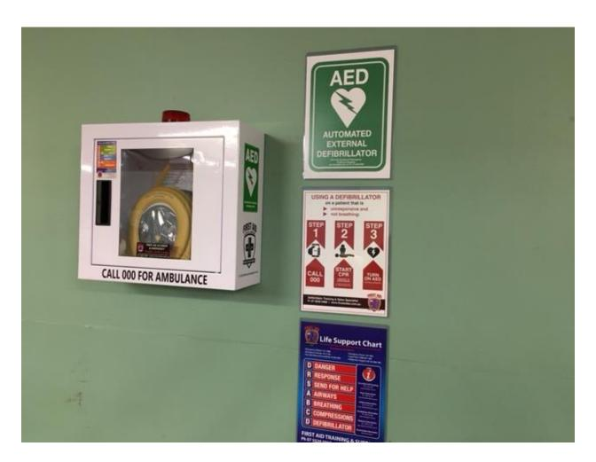
The photo is of the one in the table tennis centre in Kingston. The red light on the top of the white box fixed to the wall flashes and makes a loud noise when the door is opened.
