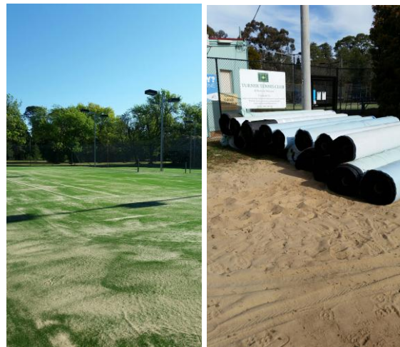
Photo: Resurfaced courts and the work in progress.
