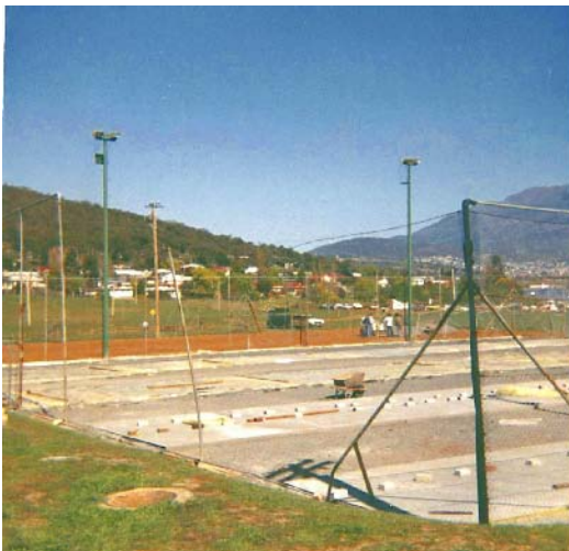
Resurfacing with no-fines
